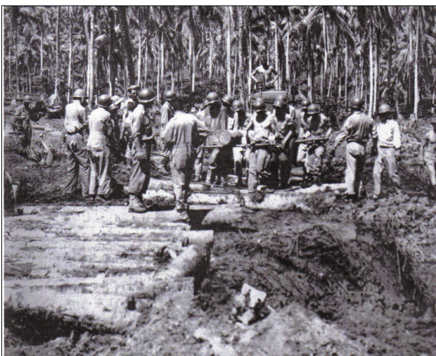
A log road is made through the jungle mud on Rendova Island. Coconut palms felled along the route served as a ready supply of road building material. Heavy artillery of the Marines was carried over this road to a point where it was in range of the Jap stronghold at Munda.
