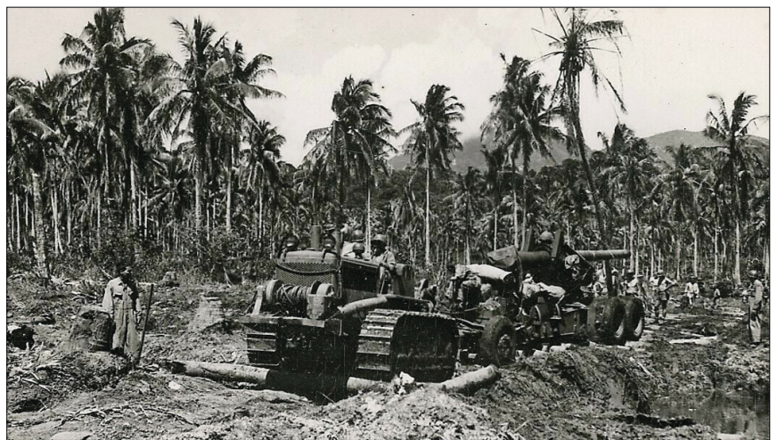
A log road is made through the jungle mud on Rendova Island. Coconut palms felled along the route served as a ready supply of road building material. Heavy artillery of the Marines was carried over this road to a point where it was in range of the Jap stronghold at Munda.
